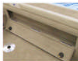
192 Port Rod Storage
